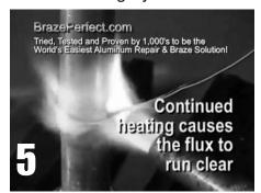
YOUR KEY TO SUCCESS! Continued heating causes the flux to change from gray to run clear. That's your signal that the repair metal is at the correct temperature to add filler alloy!
